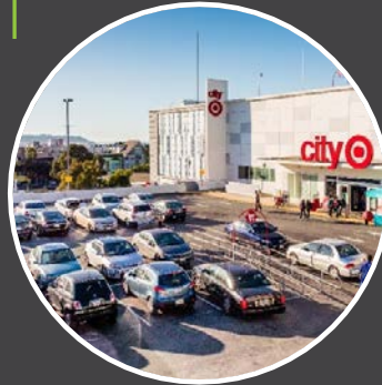
SAN FRANCISCO City Center Value-add in progress
