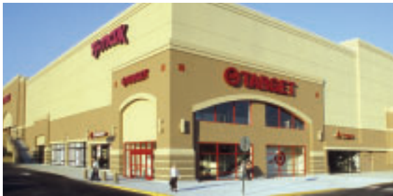
Abington Towne Center, Philadelphia, PA Multi-level 157,000 square foot Target.
