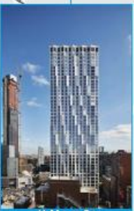
11 Hoyt St 481 Apartments
