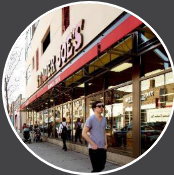
CHICAGO Clark-Diversey Value-add in progress
