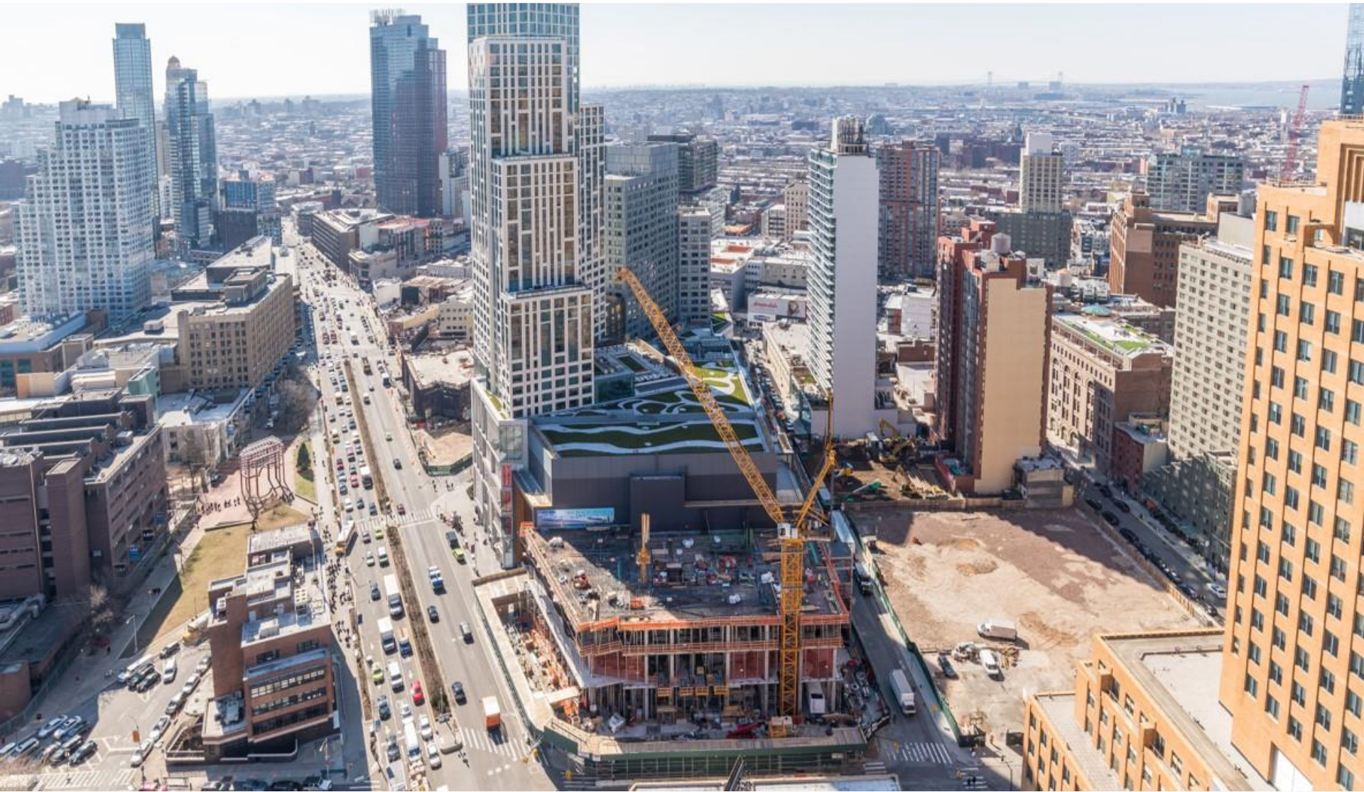
CITY POINT, CURRENT AERIAL VIEW OF GOLD ST
