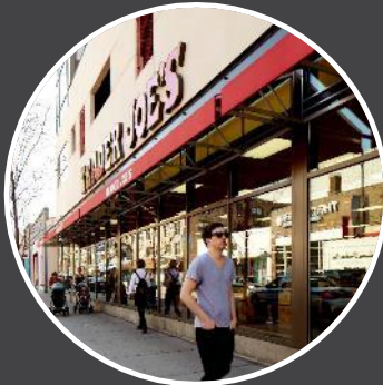
CHICAGO Clark-Diversey Value-add in progress
